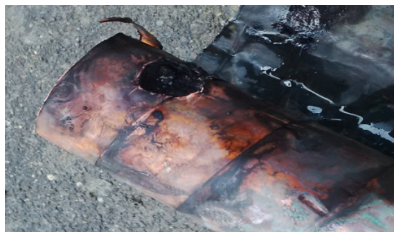
Fig.1. Irreversible partial discharge followed by breakdown of a medium voltage cable [16]
