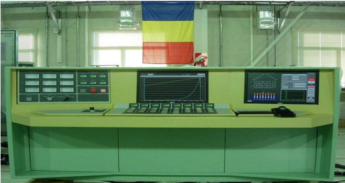
FIG. 3.15. The new TRIGA SSR 14MW operating console
