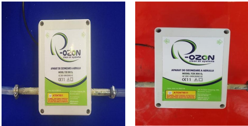
Fig. 6.4. Plan view of the pipeline-connected ozone generator [15]
