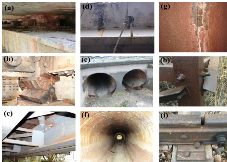
Figure 2. 5. Typical examples of corrosion defects in different parts of cast iron and steel railway structures exposed to the atmosphere: (a-d) supports, beams and bridge elements; (e-g) channel components; (h) catenary and (i) track elements [116].
