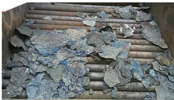
Figure 5. 5 Deposition of adherent substances on the pipe bundle of exchanger 120 S1H - general appearance
