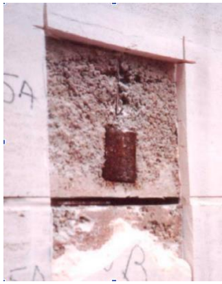
Figure 2.3. Corrosion of steel anchor plate embedded in precast concrete wall [71].
