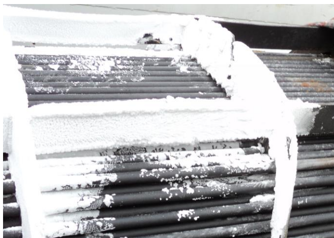
Figure 5. 9 Macroscopic appearance of deposits formed on heat exchanger elements.
