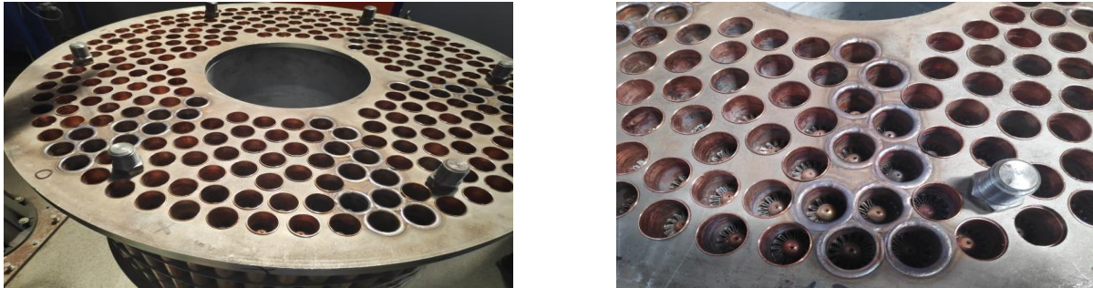
Figure 21 – Grouping and welding of sections of 10 pipes on the tubular plate
