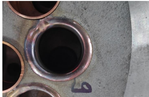
Figure 12 – Image of robotic welded areas in the case of the copper pipe with reference 9 within the heat exchanger test piece
