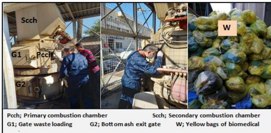
Figure 3.14 The shape of incinerator and biomedical waste[33].
