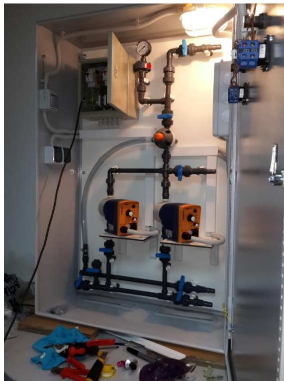
Fig. 3.3. Soda dosing facility
