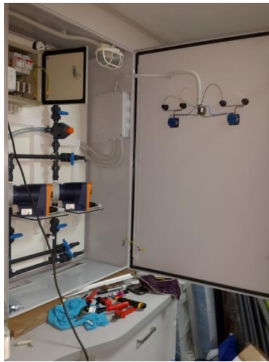
Fig. 3.4. Soda dosing facility
