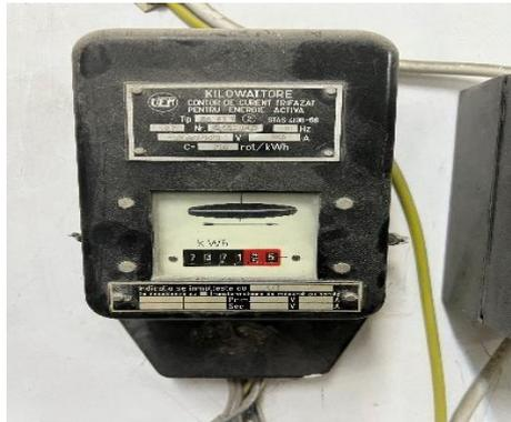
**Fig.6.10** Electromechanical meter
