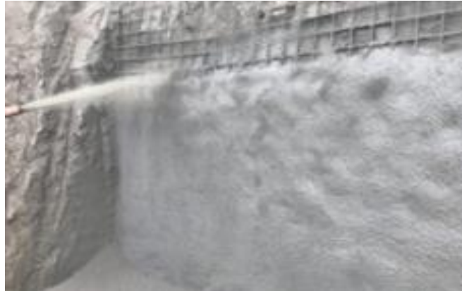
Fig. 5.4. Shotcreting procedure used to reinforce a supporting structure
