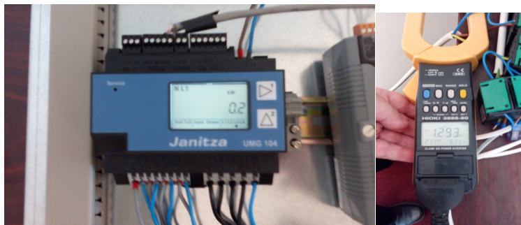
The power indicated by wattmeter W1 : P1s = 0,2kW \rightarrow P1 = 1,2 \text{ kW} The power indicated by standard P1 = 1,293 \text{ kW}
