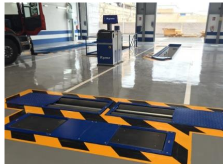
Fig. 3.7 Brake system testing stand [66]
