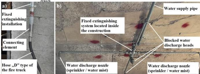
**Fig. 4.3.** Fixed extinguishing system located: a) outside the test room, perpendicular to the wall with the door; b) inside the test room, at the ceiling
