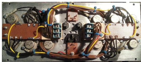
Fig. 2.2 Power supply transistors connected on the heatsink
