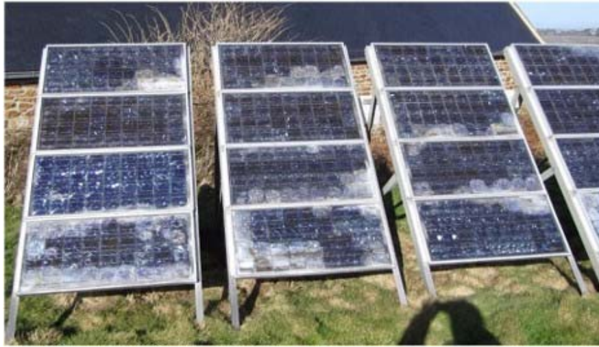
Fig. 3.1 Salt deposits on the surface of pv panels in maritime climate[5]
