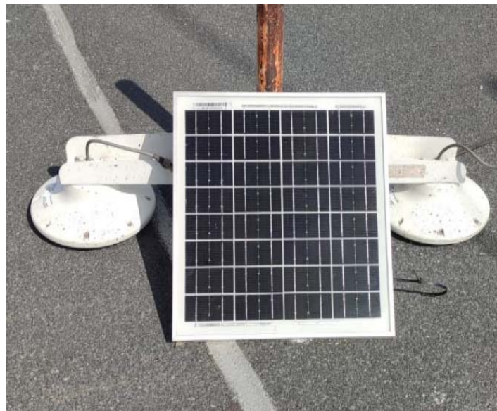
Fig. 5.3 Installation of the PV panel on the building of the Faculty of Marine Engineering
