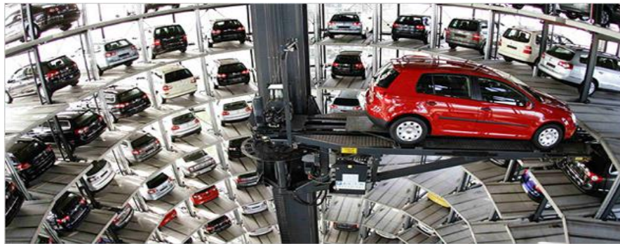
Fig. 3. Moving a vehicle vertically by the elevator inside the parking lot
