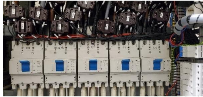
Figure 6.3 Installation of Current Transformers
